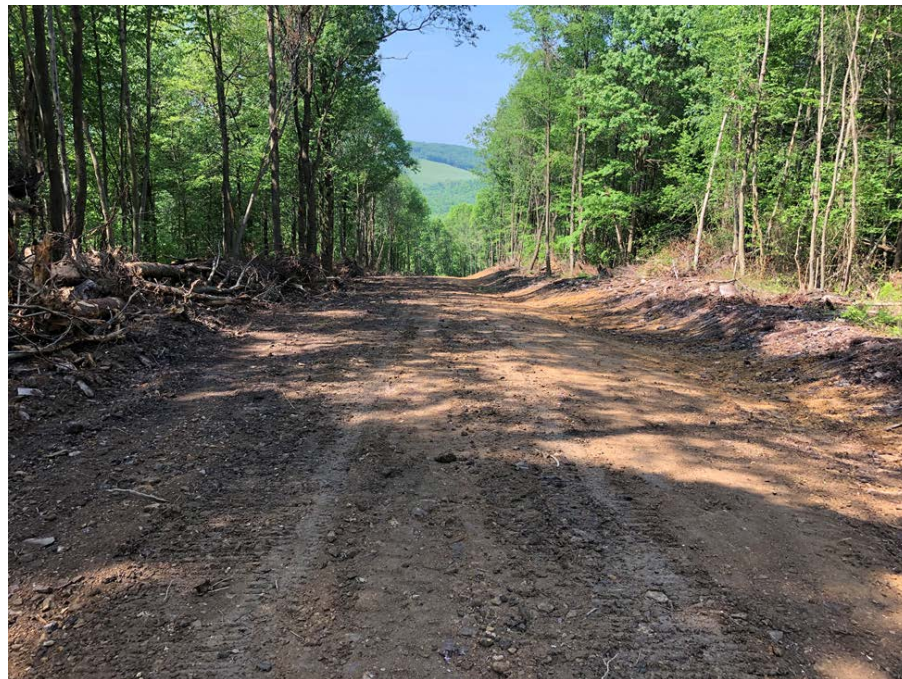
DETAIL – ROAD SECTION GRADED AND ROLLED PRIOR TO BASE STONE APPLICATION
